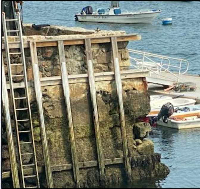
Parker Boat Yard seawall
