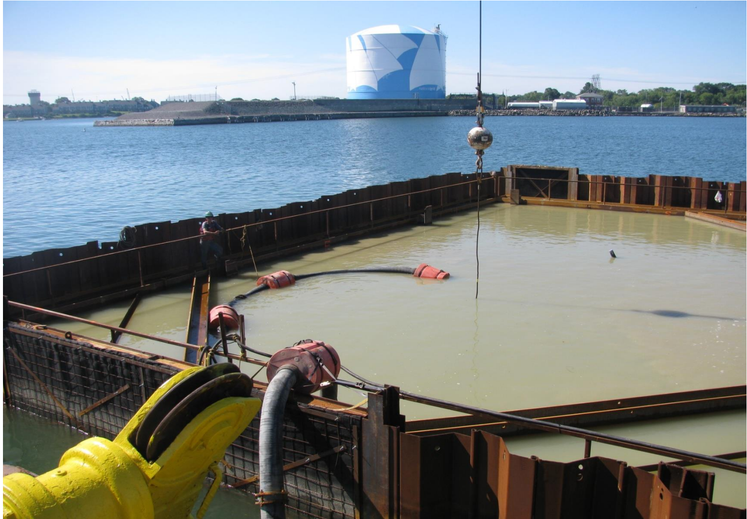
Dredging and HDD within a cofferdam
