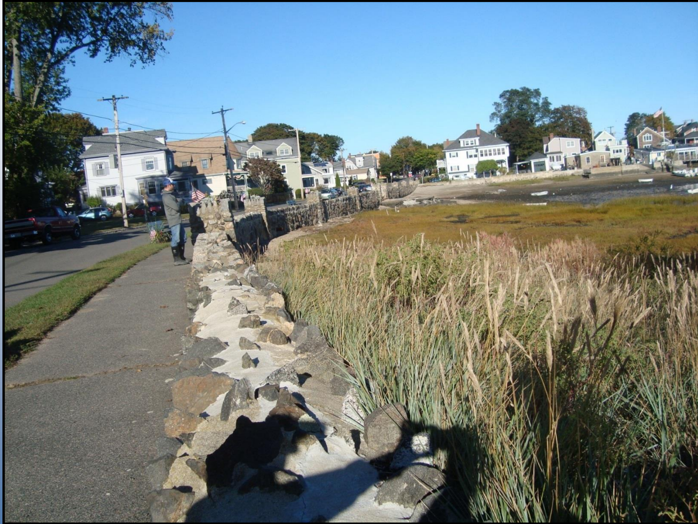
Columbus Avenue, sidewalk and low retaining wall next to marsh.
