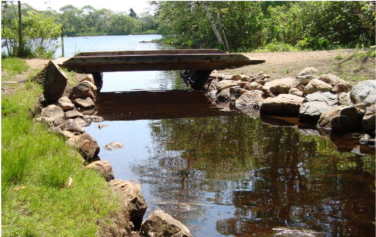
Figure 3. New footbridge replaced in 2011 at Clark Pond
