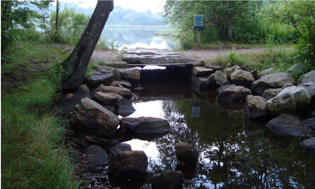
Figure 2. - Pre-construction: culvert and footbridge tidal restriction at Clark Pond
