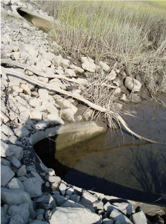
Two culverts discharge water into the marsh.
