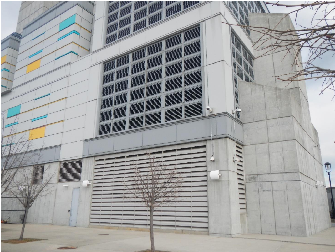
Vent Building 1 – Detail of Air Exchange Vent
