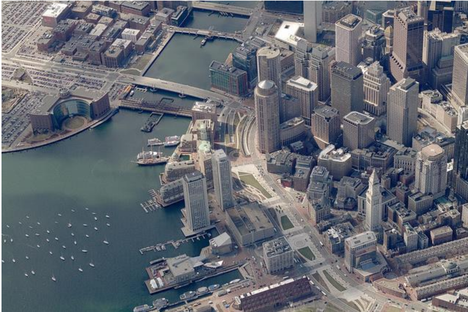
Boston Harbor & Tip O'Neill Tunnel Exit/Entrance Ramps http://www.flickr.com/photos/pictometry/6220376808/
