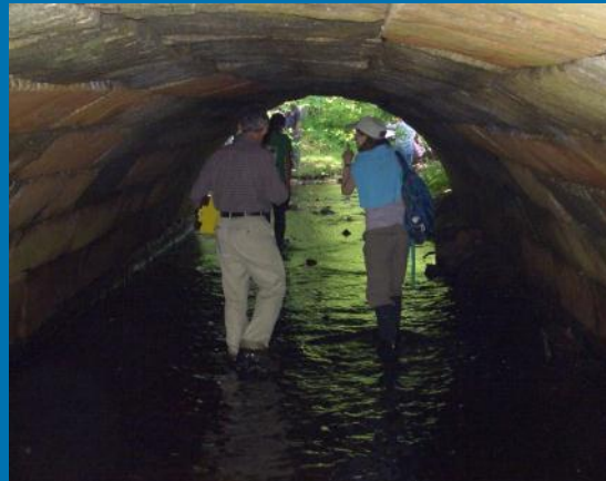
Assess adequacy of culvert sizes
