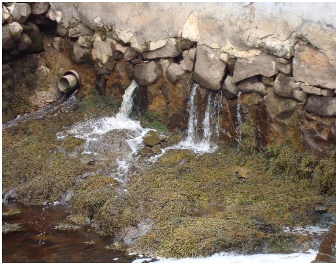
Central Street Bridge/Tidal Gate
