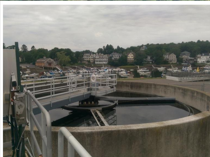
Wastewater Treatment Plant
